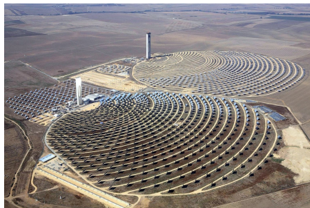
Solar Power Plants
