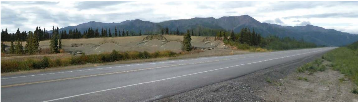
d. Existing Winter Conditions
