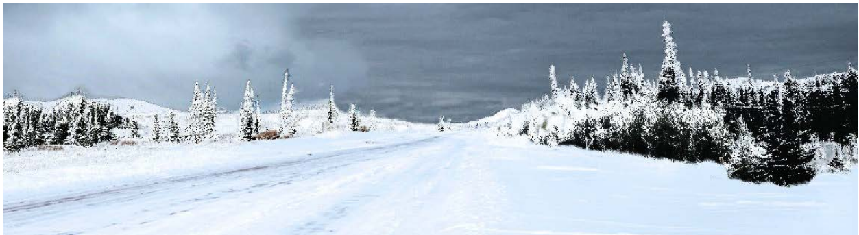
e. Winter Conditions After Construction
