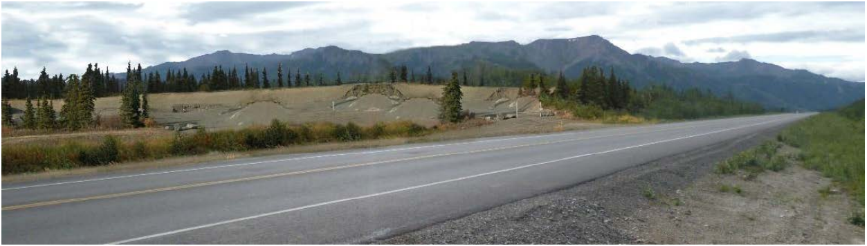
c. After Construction
