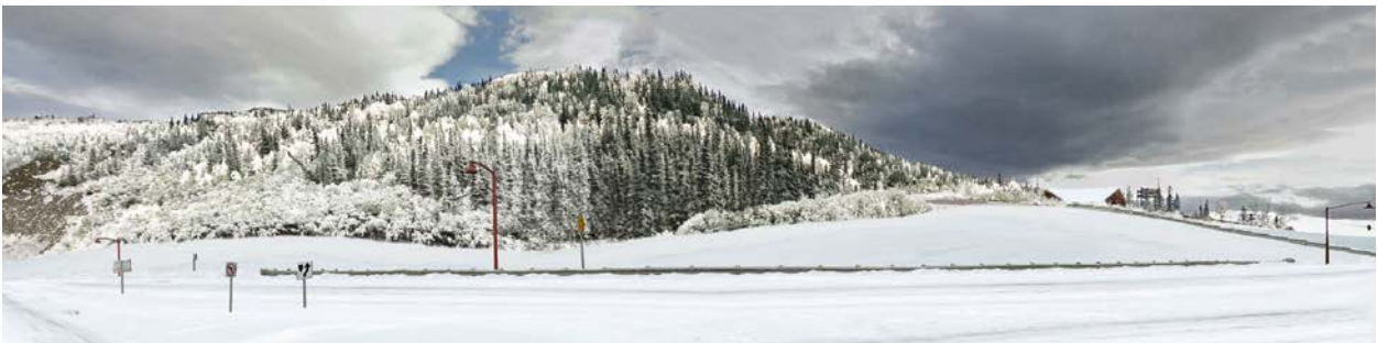
e. Winter Conditions After Construction
