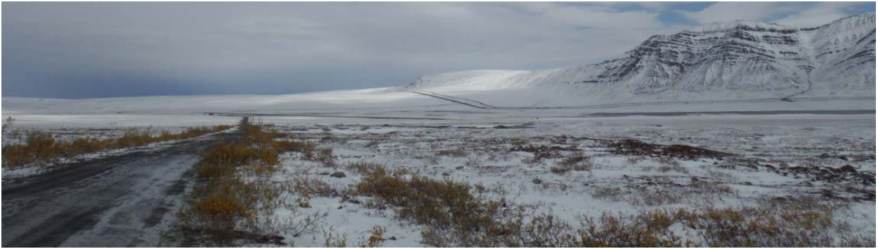
c. After Construction
