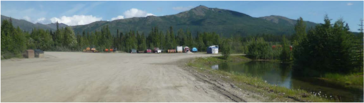
c. After Construction
