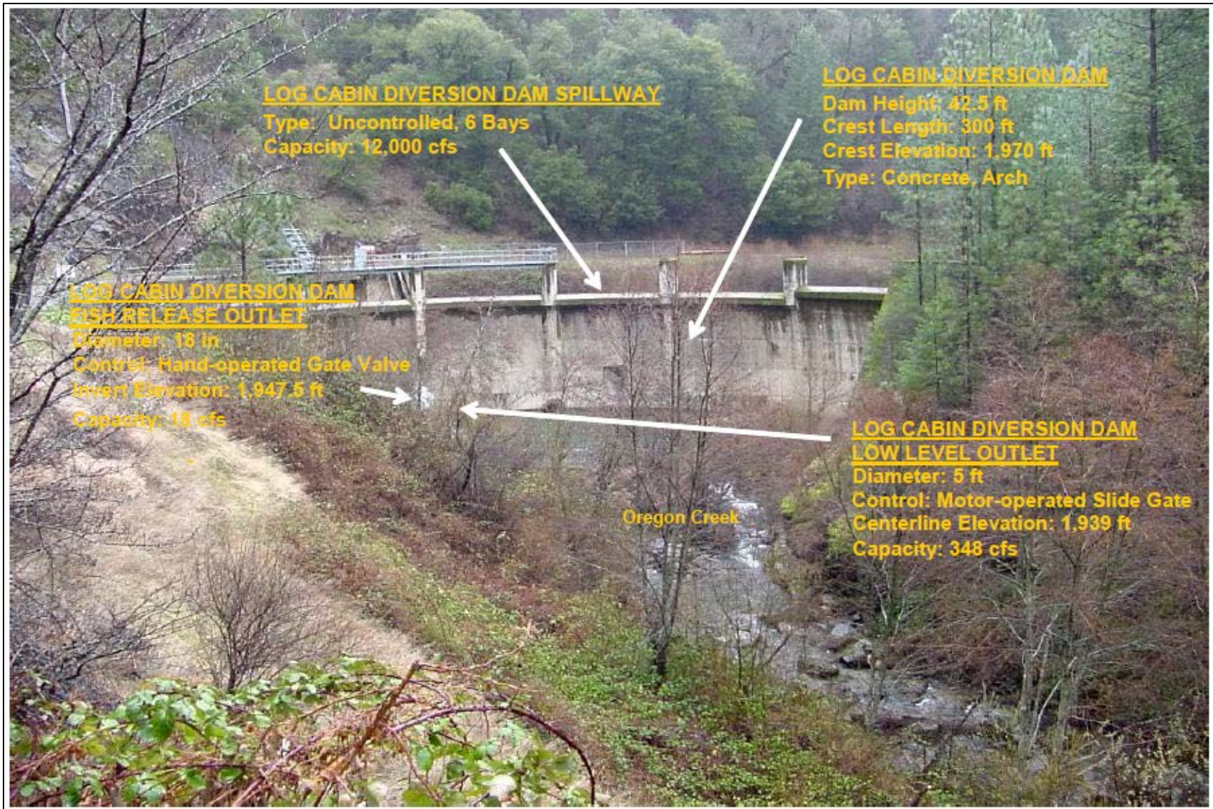
Figure 2-2. Log Cabin Diversion Dam (Source: YCWA, 2017a).
