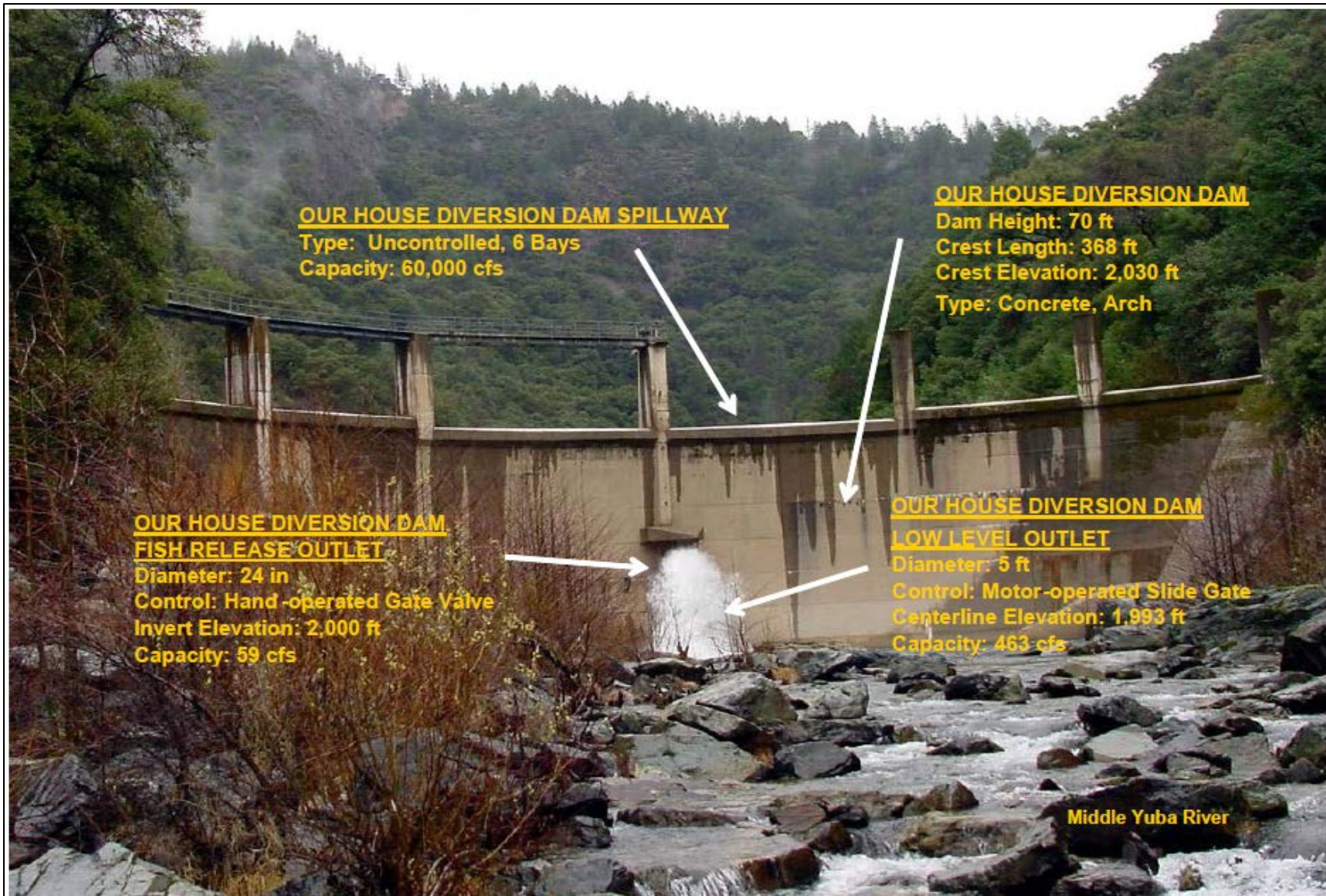
Figure 2-1. Our House Diversion Dam (Source: YCWA, 2017a).
