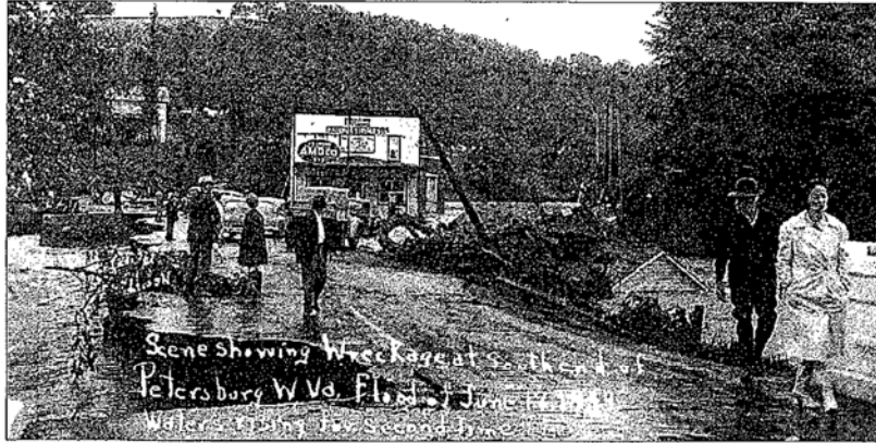
The 1949 flood hit region-wide in Virginia and West Virginia, nearly mimicking the flooding that occurred in 1985. This photo, from the Kent Botkin collection, depicts the damage at the southern end of Petersburg, W. Va., following that storm.
