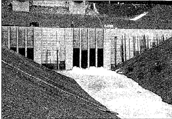
Water arrives at the upper reservoir during a test on the generators as pumps. Engineers on the project were caught by surprise when the remnants of Hurricane Juan filled the lower reservoir in only 24 hours, instead of 10 months, as planned. (Photo courtesy Robin Sullenberger)
