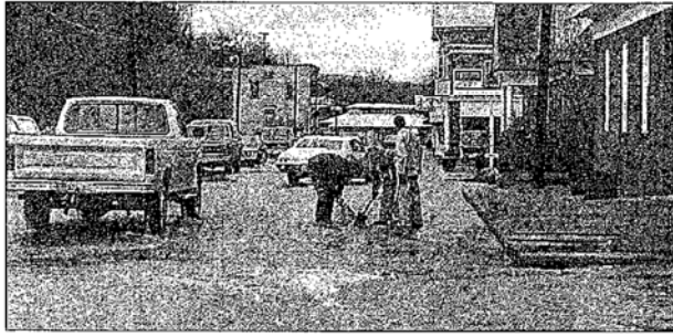
Hot Springs residents jumped in to unclog storm drains to lower the water level on Main Street. The creek behind the businesses on the right overflowed its banks, and washed down the street and into most of the establishments during 1985's flood. (Recorder file photo)
