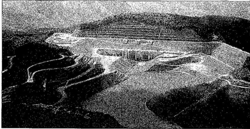
The Bath County Pumped Storage Station was very near completion in 1985, following years of construction and planning. Engineers tested the generators and pumps, and used them to fill the upper reservoir from below. Here, the water in the upper reservoir was still well below full height level prior to the flood of 1985. (Photo courtesy Robin Sullenberger)
