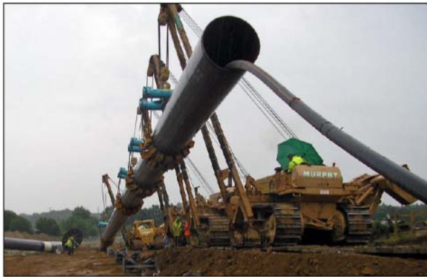
FIGURE VII(f) – Final section of pullback pipe for an HDD operation in relatively flat terrain.
