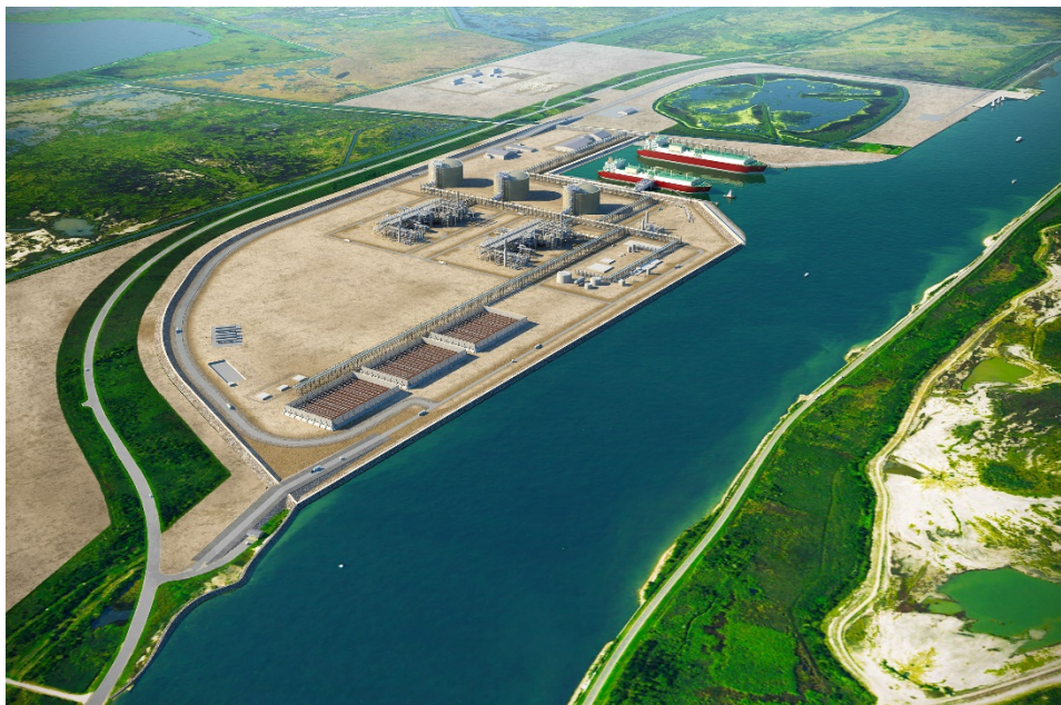
Source: Semptra LNG & Midstream, Port Arthur Liquefaction Project Website, 2018
