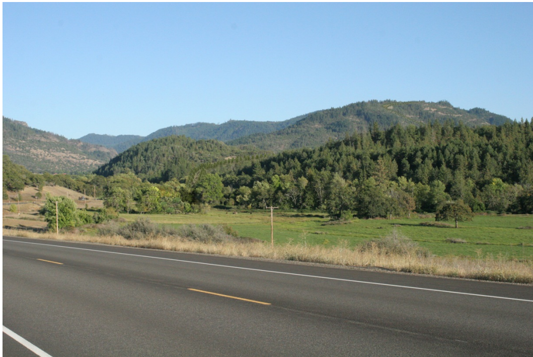
Figure 4.8-19b. KOP-P3. Highway 140 near Little Butte Creek (MP 145.6). Simulated views of the pipeline right-of-way as viewed from the Highway 140 crossing, at 5 and 25 years following construction, respectively.
