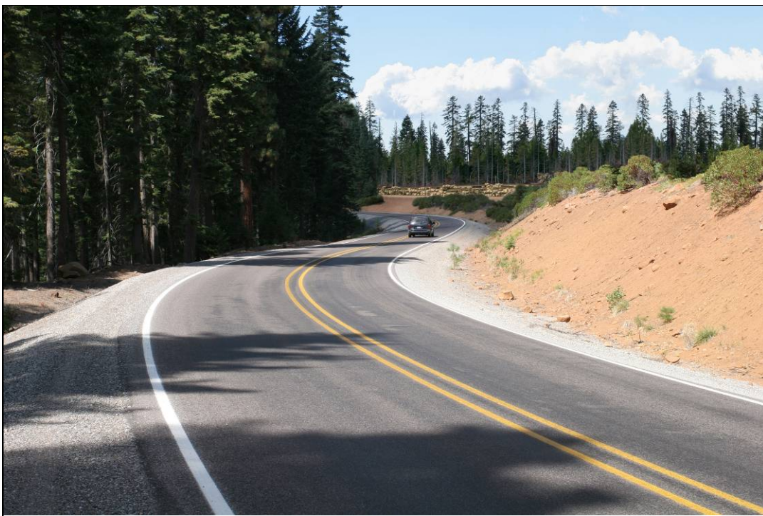
Figure 4.8-22a. KOP-P6. Clover Creek Road (MP 176.8). Existing (above) and post-construction simulation (below), of the pipeline right-of-way as viewed from Clover Creek Road near Spencer Creek.
