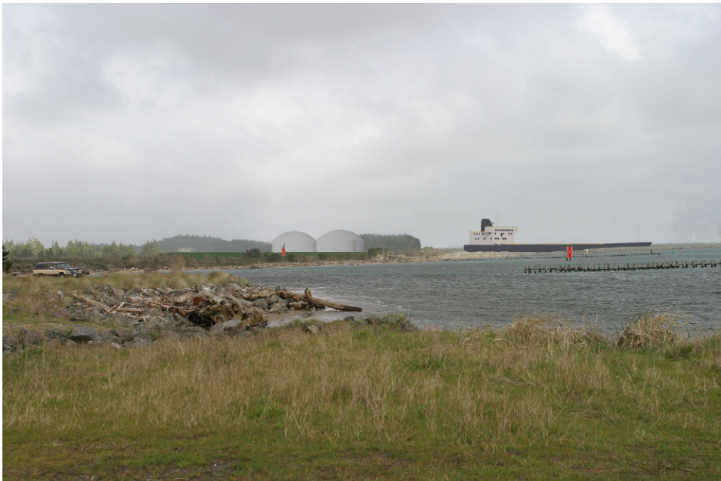
Figure 4.8-13. KOP-T11. BLM North Spit Boat Launch Area. Existing and simulated views of the LNG Terminal from the BLM North Spit Boat Launch Area, on the North Spit.
