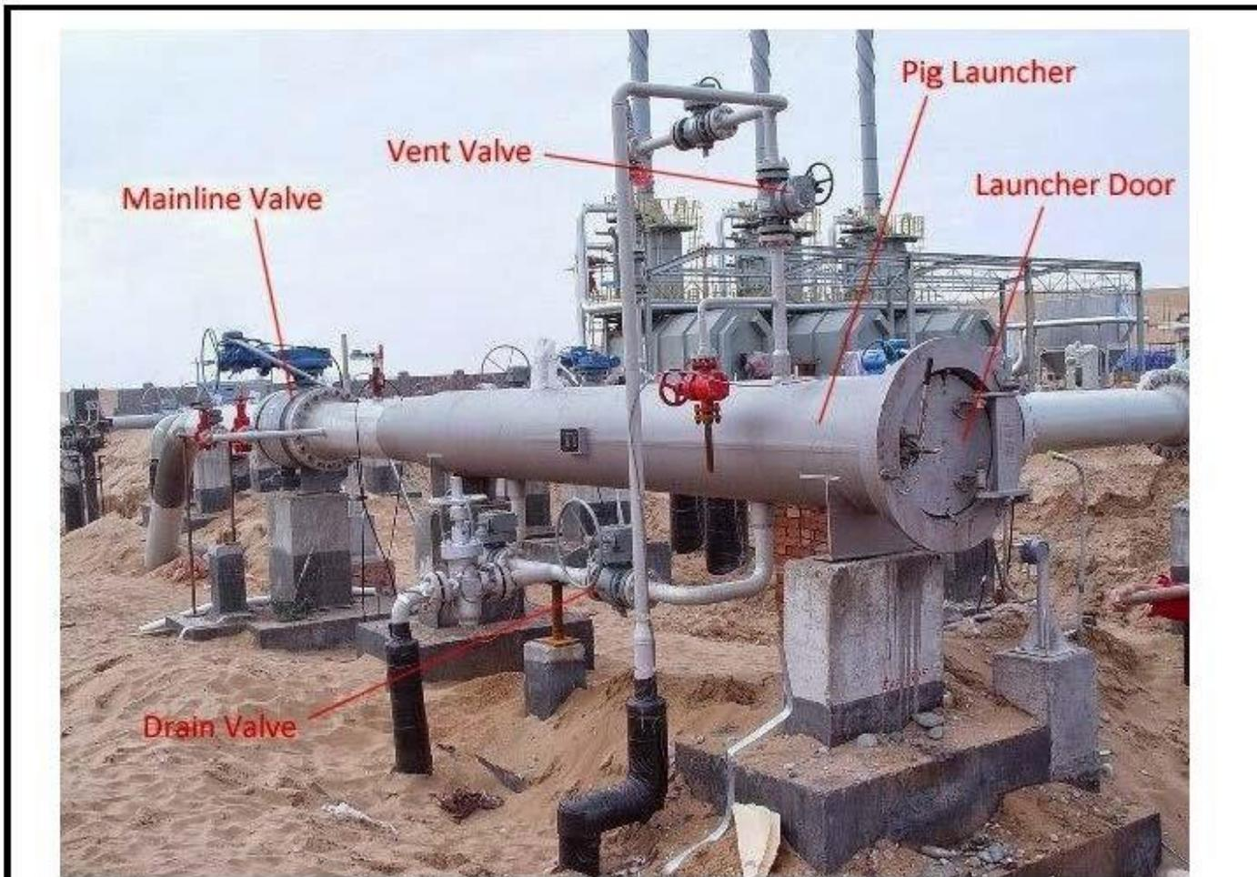
Typical Pig Launcher and Receiver
