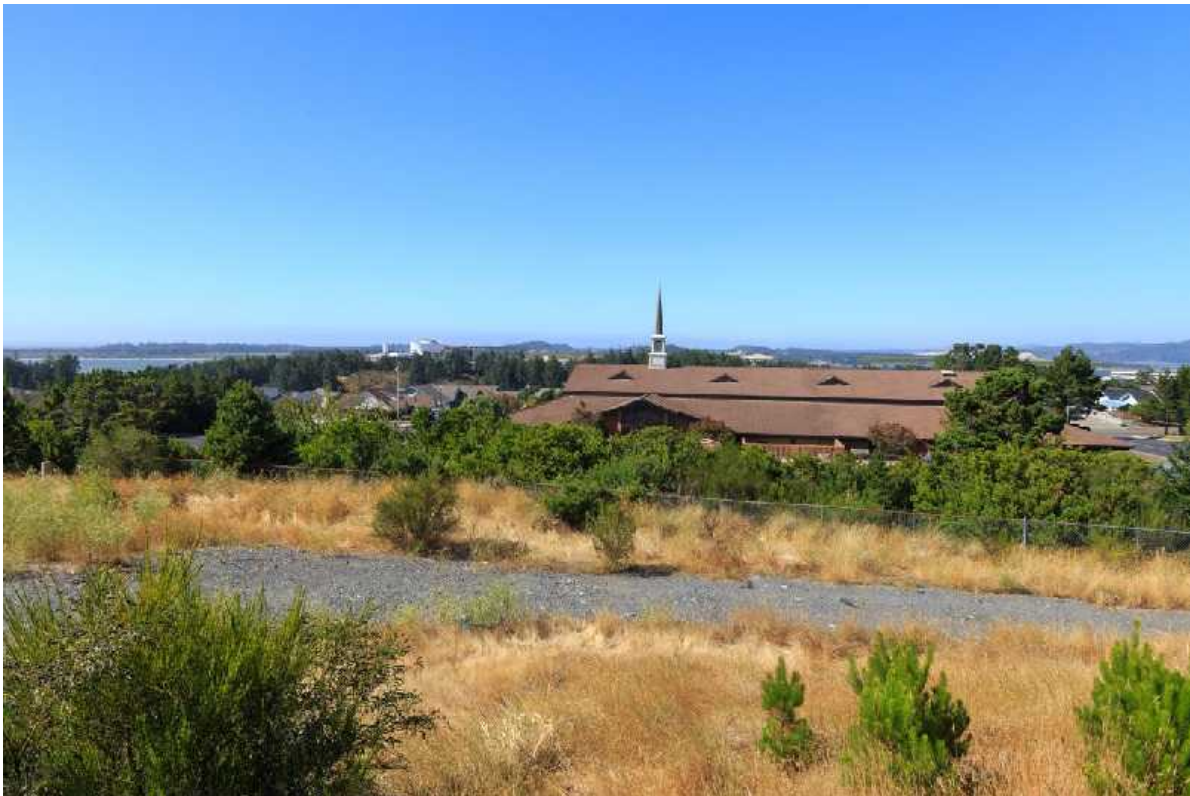
Figure K-9. Viewpoint-9. North Bend, Open Space near Washington Avenue. Existing view and simulated view of the LNG terminal site, marine slip, and concrete perimeter walls.
