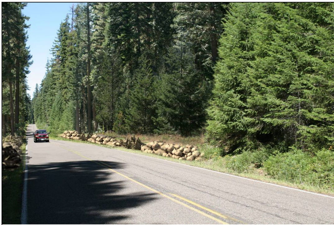
Figure K-15b. KOP-P4. Big Elk Road (Forest Road 37, MP 161.4). Simulated views of the pipeline right-of-way as viewed from at the Big Elk Road (Forest Road 37) crossing, at 5 and 25 years following construction, respectively.
