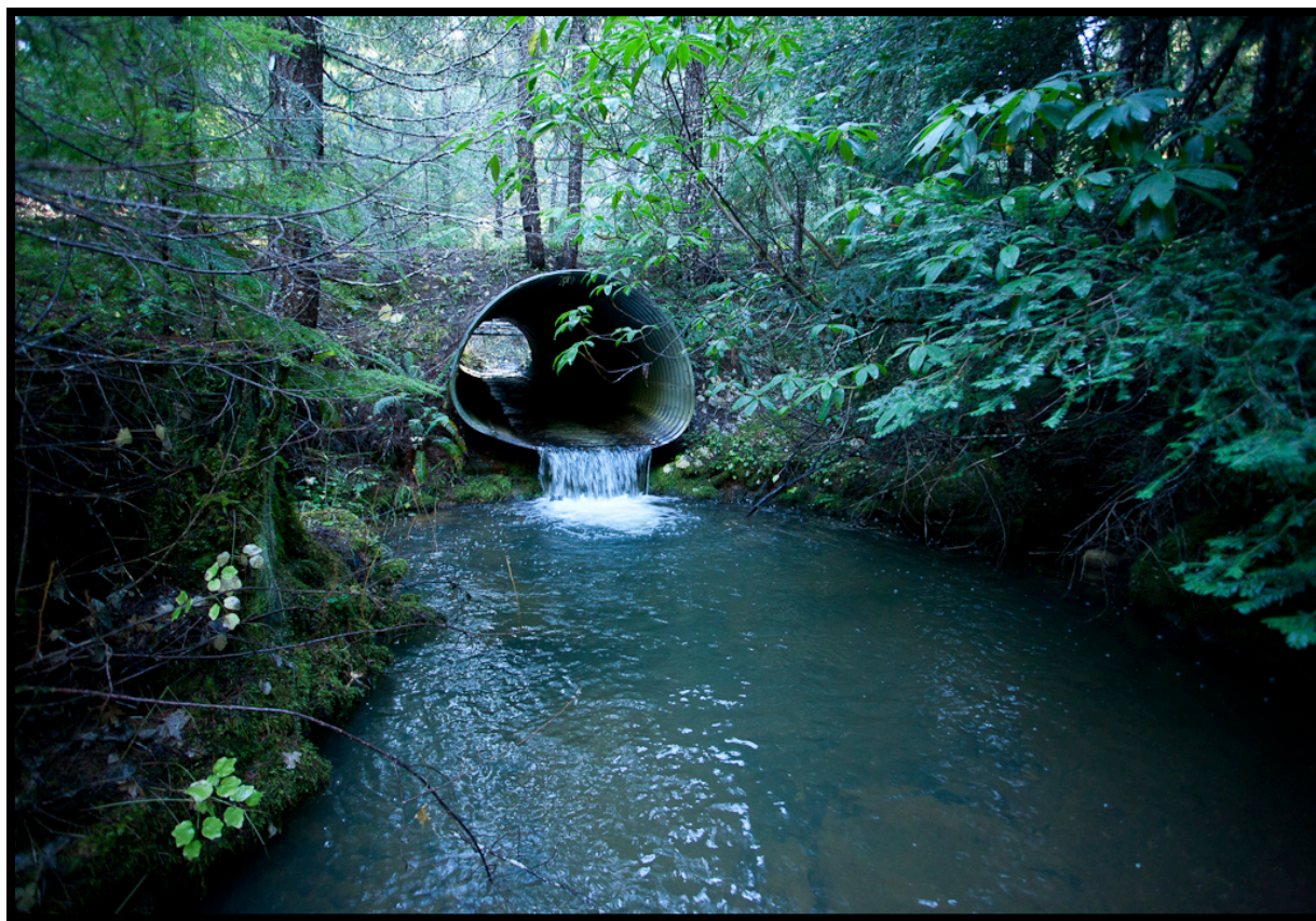
Figure 2-8 East Fork Cow Creek Culvert. This culvert currently blocks migration of fish and other aquatic biota. It would be replaced by a “fish-friendly” design as part of the mitigation plan proposed by Pacific Connector.
