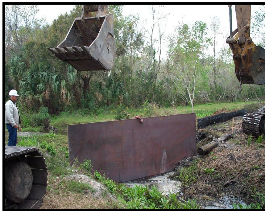
Figure 1-3 Installation of a dam in a dry open cut crossing of a small channel
