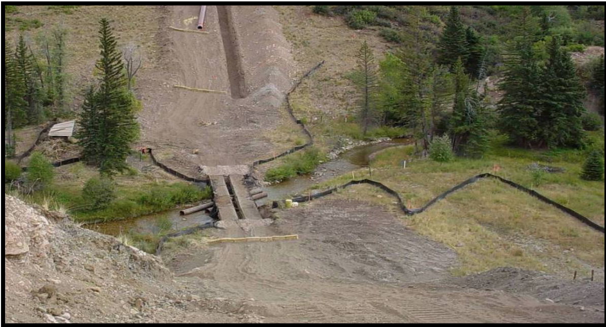
Figure 1-5 Dam-and-pump crossing of perennial stream with flume.
