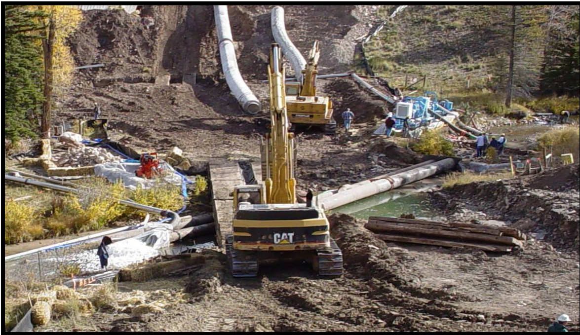
Figure 1-5 Dam-and-pump crossing of perennial stream with flume.
