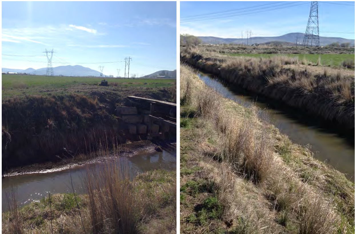
Crossing 1, No. 1 Drain looking east (left image) and north (right image)
