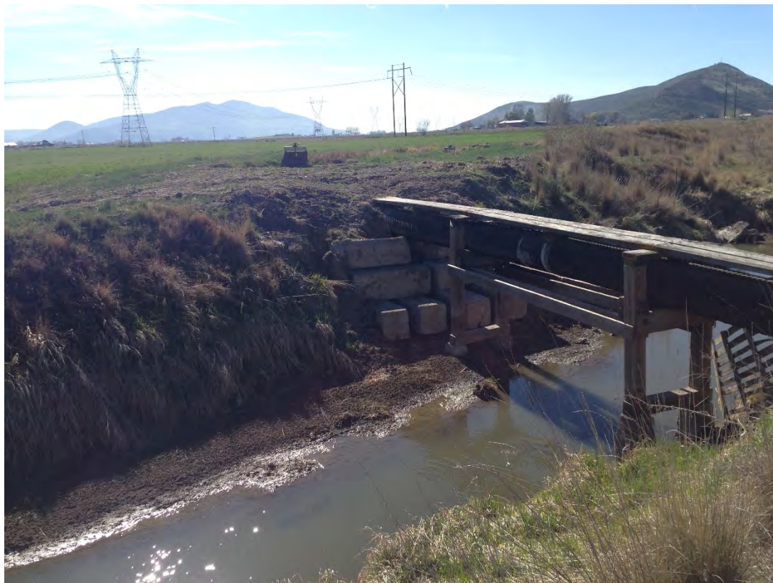
Crossing 1, No. 1 Drain looking southeast
