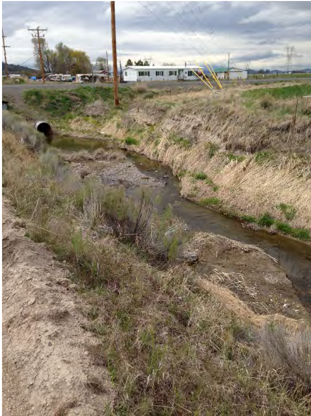
Crossing 18, No. 5 Drain looking west
