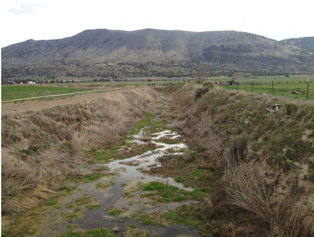
Crossing 19, 5-H Drain looking northeast
