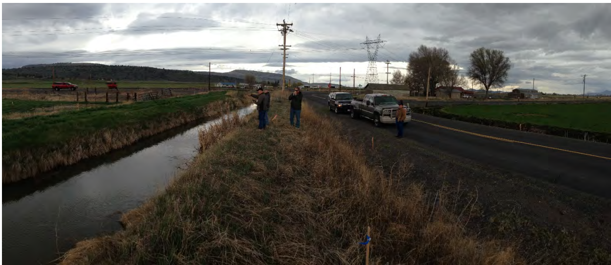
Crossing 17, C-9 Lateral panorama looking west, Matney Way to the right
