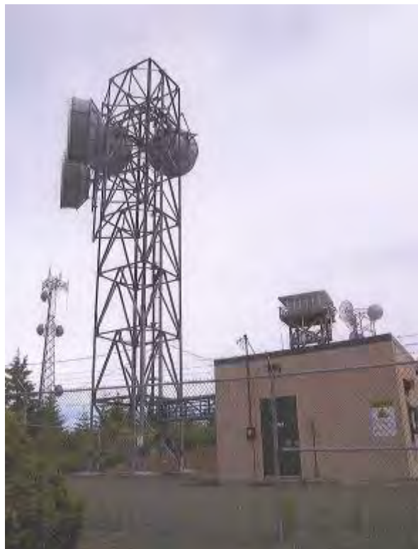
Photo 2. American Tower Site at Signal Tree (Kenyon Mtn.)
