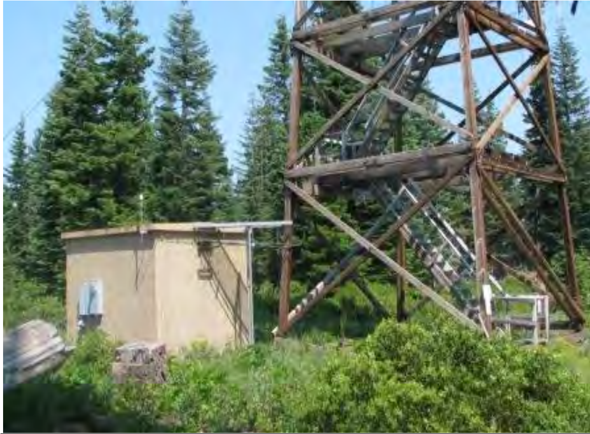
Facility 1 – US Cellular
