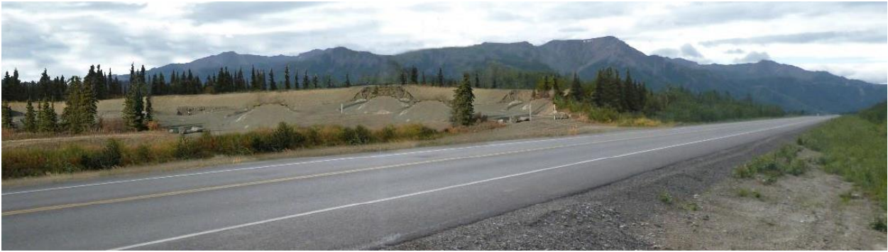
c. After Construction
