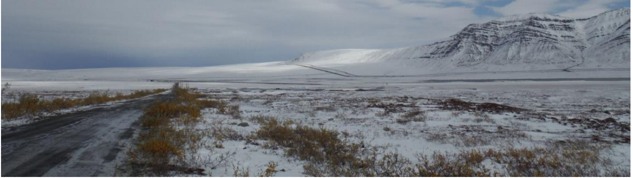
c. After Construction
