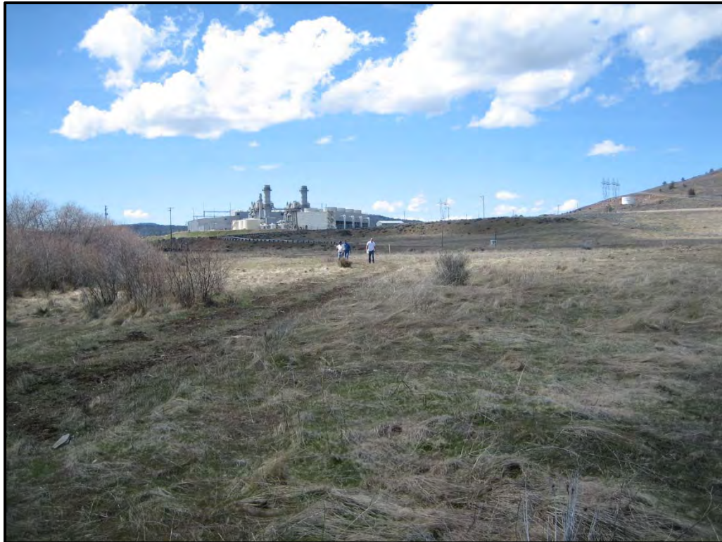
Looking West Towards Pipe Stringing and Fabrication Workspace
