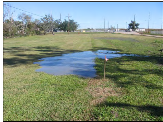
Photograph 1 - Example of Drilling Fluid Surface Release
