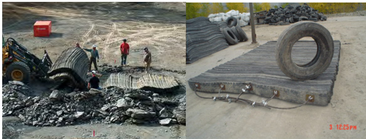
Photo 1 Typical Blast Mats Made from Used Tires
