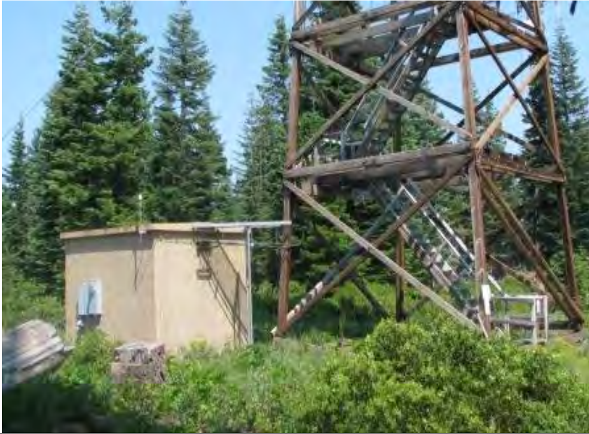
Facility 1 – US Cellular
