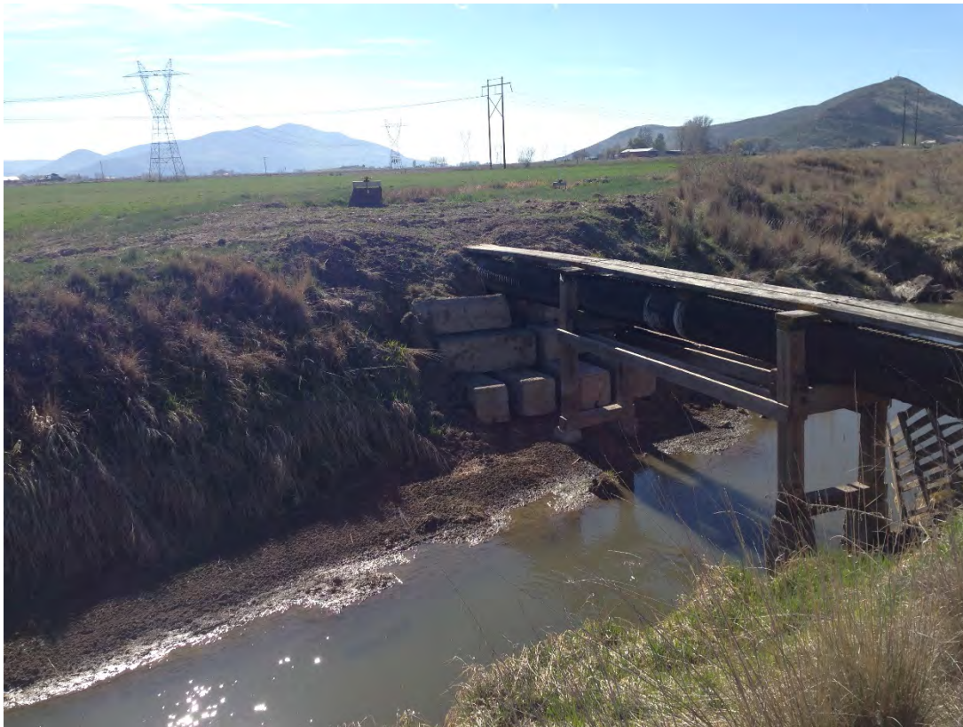
Crossing 1, No. 1 Drain looking southeast
