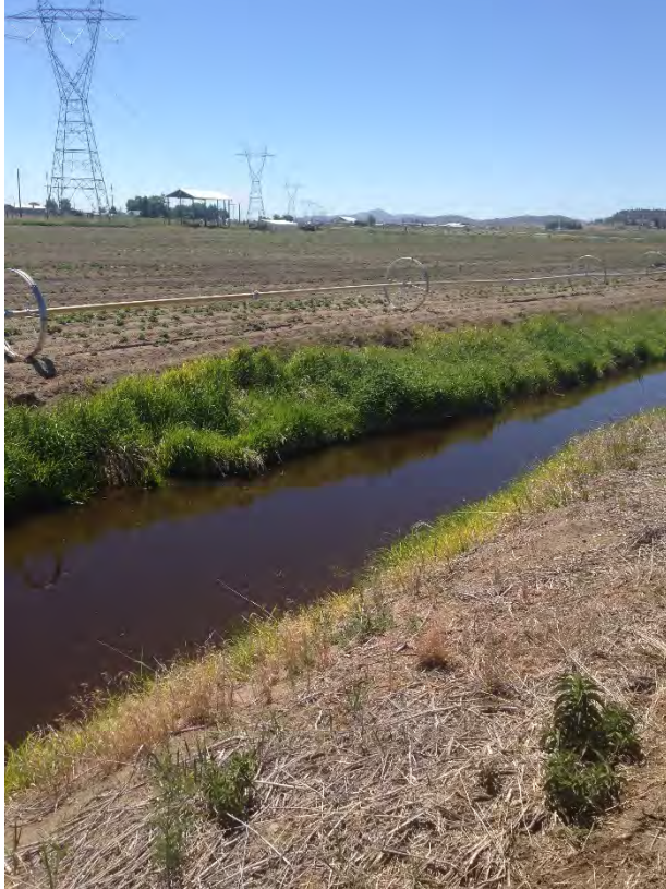
Crossing 15, 5-A Drain looking southeast
