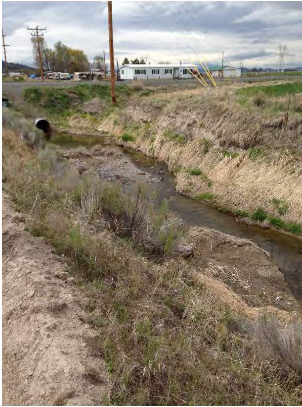
Crossing 18, No. 5 Drain looking west
