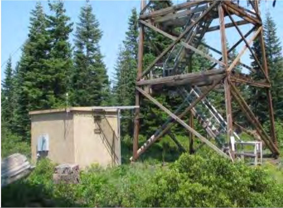
Facility 1 – US Cellular
