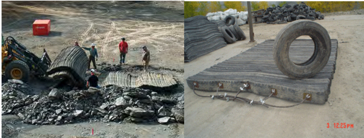
Photo 1 Typical Blast Mats Made from Used Tires
