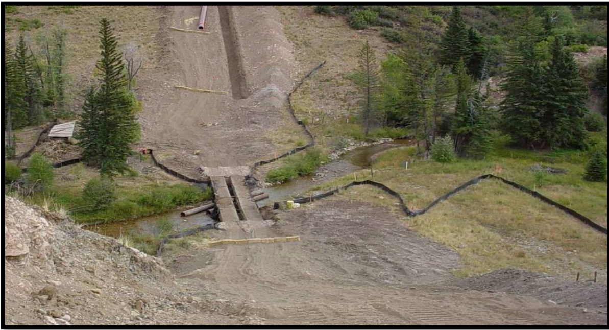
Figure 1-5 Dam-and-Pump Crossing of Perennial Stream with Flume
