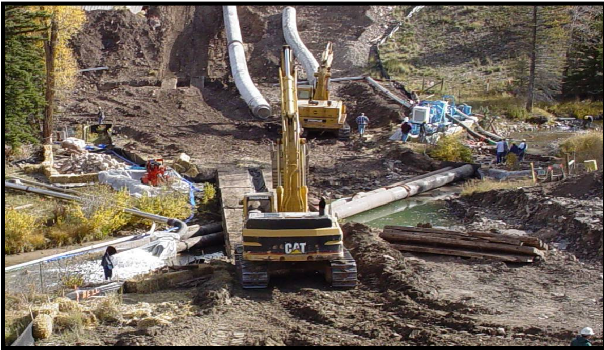
Figure 1-5 Dam-and-Pump Crossing of Perennial Stream with Flume
