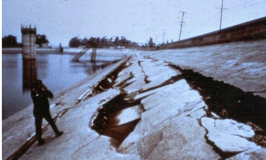
Figure 2-14 Close-up View of Cracks in the Upstream Face of Upper San Fernando Dam.
