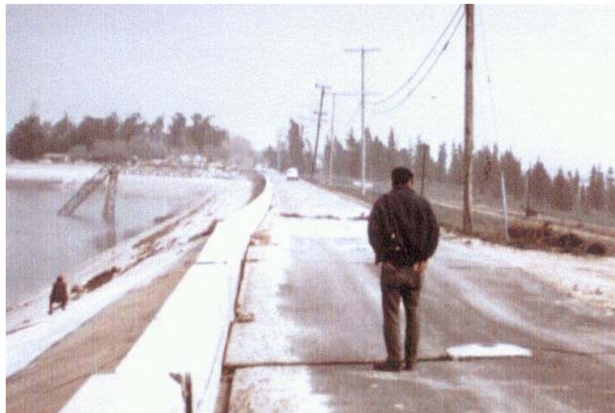
Figure 2-13 View of Upper San Fernando Dam showing horizontal and vertical deformations and cracks in the upstream face of the dam.
