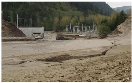
Fig. 11. Fissure at Swift #2 Power Canal.
