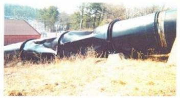
Fig. 4. Buckled steel penstock.
