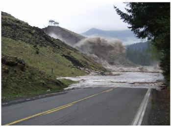
Fig. 8. Swift #2 Power Canal failure.
