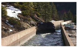
Fig. 13. Rock inside power canal.
