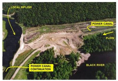
Fig. 9. Hatfield power canal failure.
