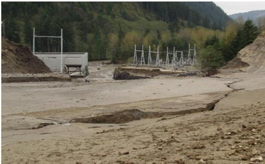
Fig. 11. Fissure at Swift #2 Power Canal.
