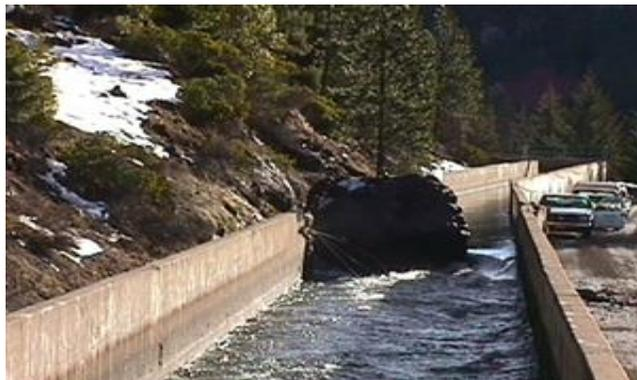
Fig. 13. Rock inside power canal.
