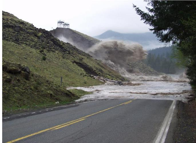
Fig. 8. Swift #2 Power Canal failure.
