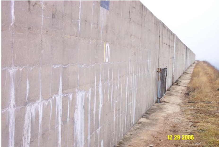
Figure 4.2 - Panel 10 Note grass is lain over near footing Damage from overtopping was judged as Minimal Estimate 0.1 ft. of overtopping
