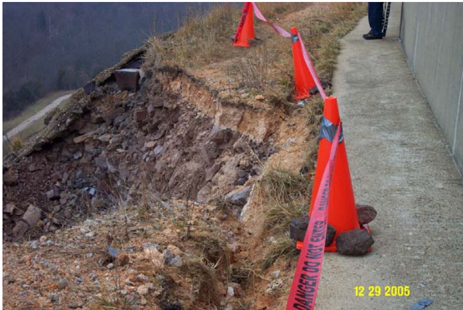
Figure 4.6 - Panels 48 and 49 Scarp near toe of parapet wall footing Note erosion rut adjacent to the footing
