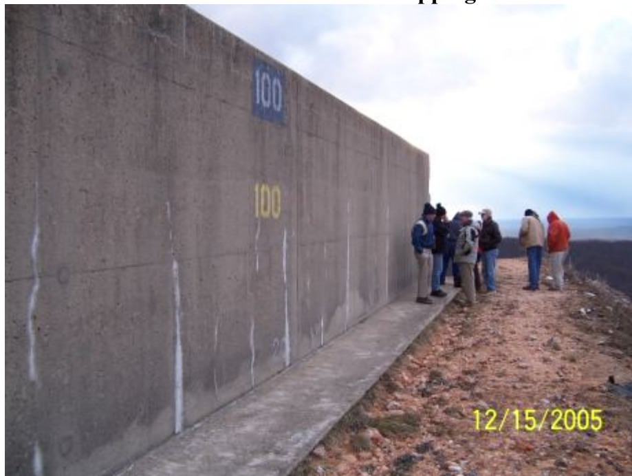
Figure 4.2 - Panel 10 Note grass is lain over near footing Damage from overtopping was judged as Minimal Estimate 0.1 ft. of overtopping
