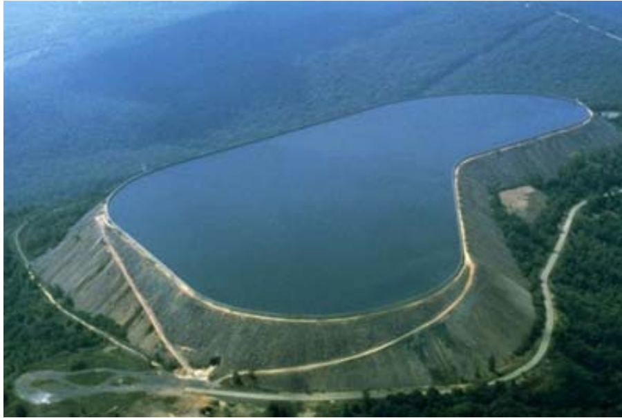
Figure 2.3 - View of upper Reservoir.
