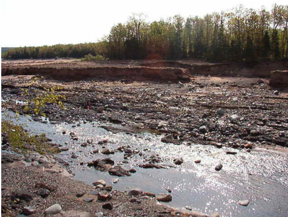
Photograph 4. View of the upstream portion of the channel as viewed from the right abutment near Station 0+35. Photograph taken on June 3, 2003.
