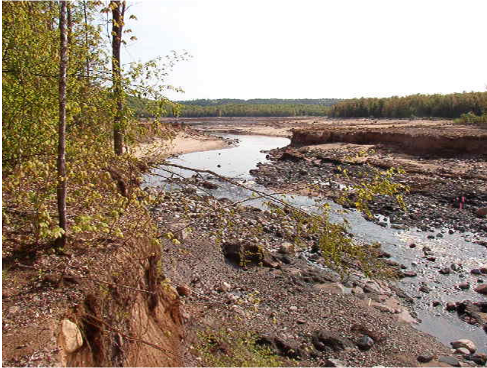
Photograph 3. Silver Lake channel entrance as viewed from the right abutment near Station 0+35. Photograph taken on June 3, 2003.
