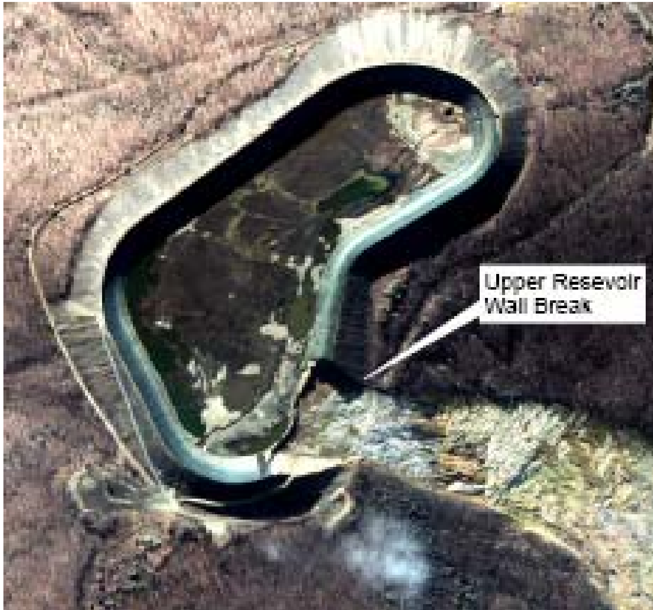
Taum Sauk Upper Reservoir Breach 12/14/05
