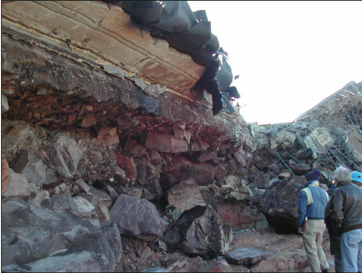
Rockfill between top of rock and base of plinth, note reddish grout in rockfill beneath the plinth
