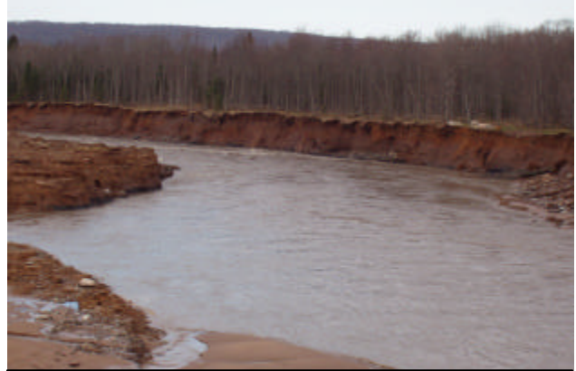
Photo 6. Erosion below Silver Lake. Source UPPCO 5/15/03
