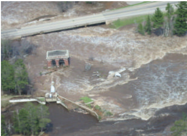
Photo 13. Tourist Park dam breach. Source MDNR 5/15/03
