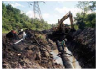
Dewatering pipeline trench
