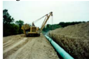
Lowering pipe in trench
