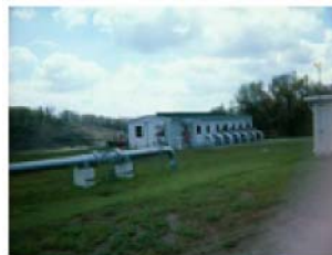
Compressor station building
